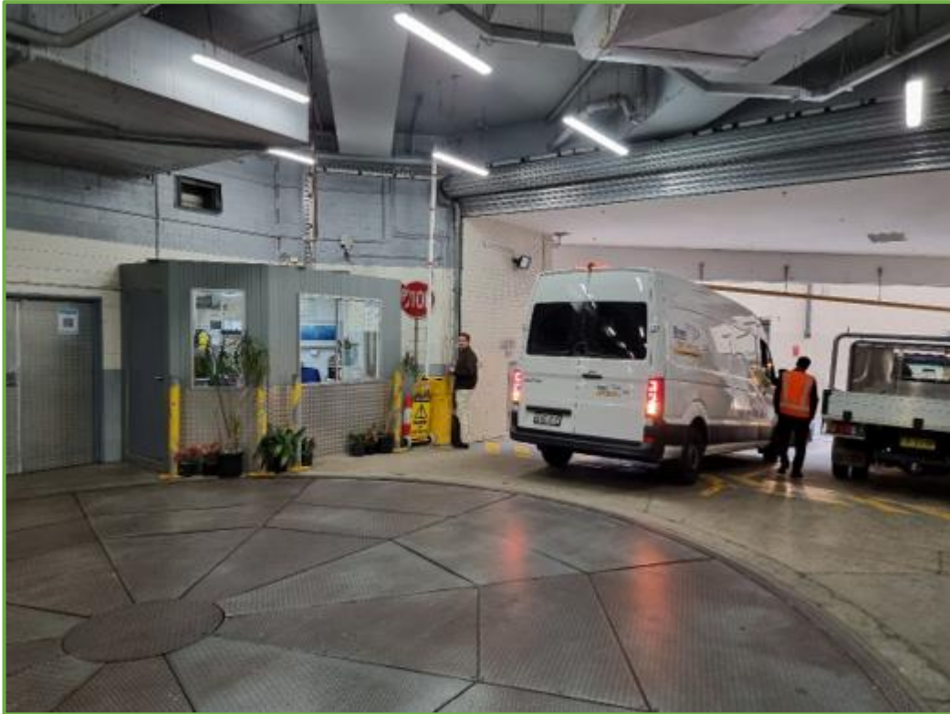
Figure 3: View looking towards the existing security office (not shown on the plans) located in the south-eastern corner of the loading dock
